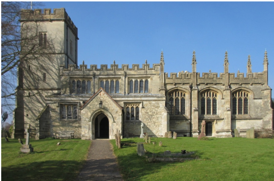
St Mary's Church, a Grade 1 listed building, is regarded as amongst the finest in the country, and was largely built with the offerings of pilgrims to the village in medieval times
